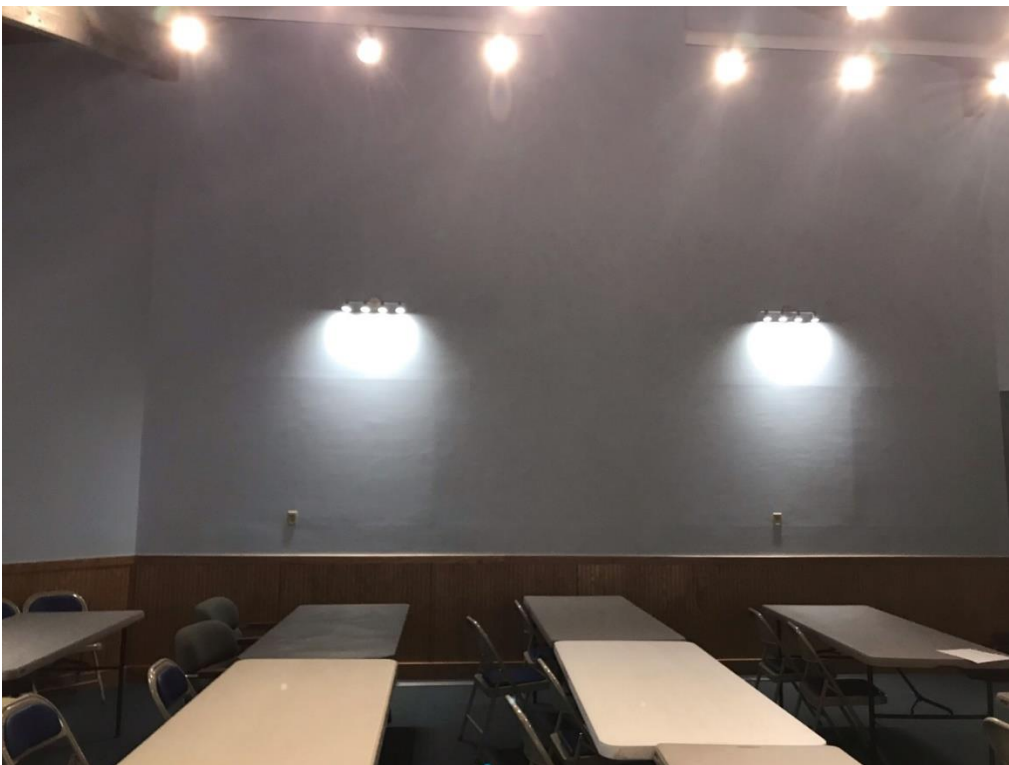
PICTURE 4 – Another view of the Lake Erie Map (#1) wall. The map will be centered under the light fixtures. The outlets will be moved lower on the wall.
