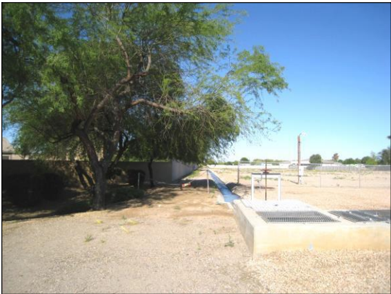
Irrigation Canal and Access Easement Along South Portion of the Subject
