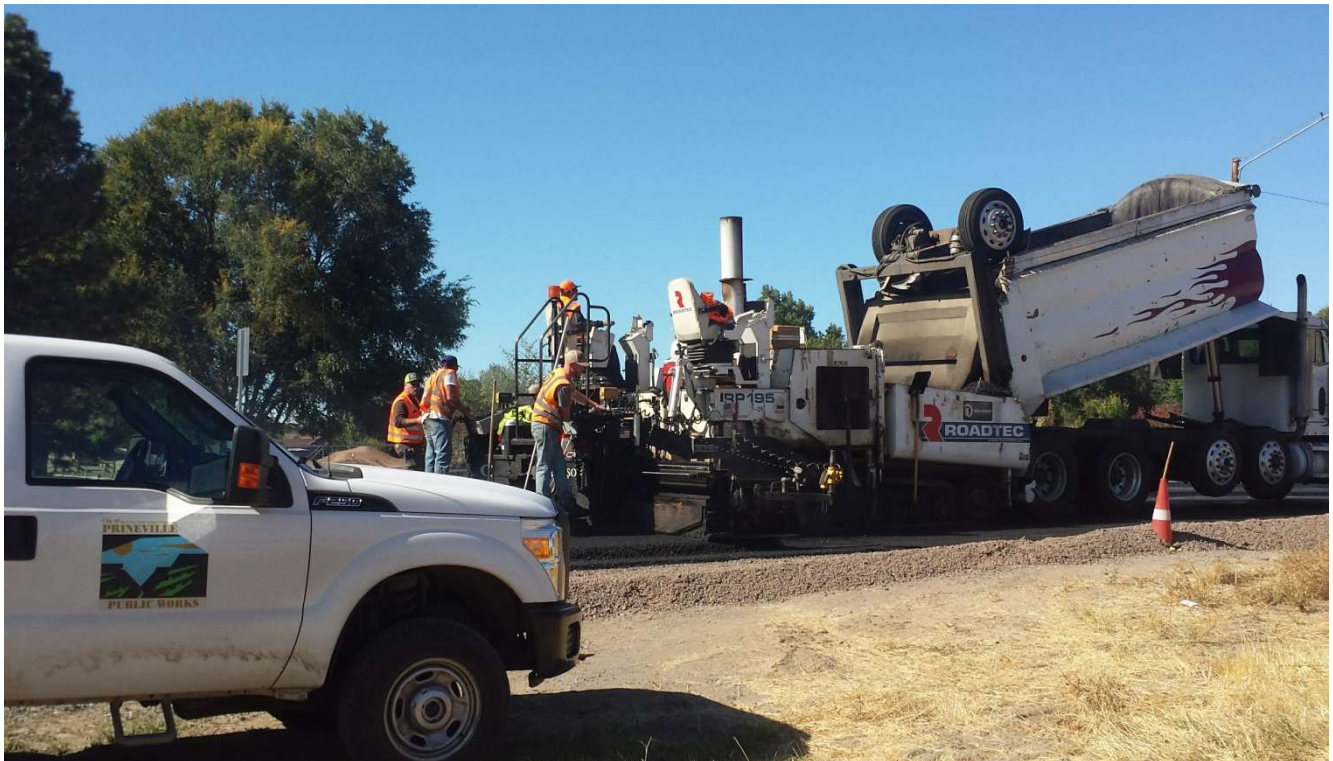
Crews work to lay down asphalt on NE Juniper Street during a paving project in October 2017.
