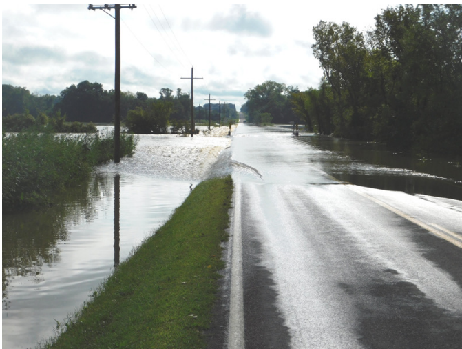
N 1000 RD flooded July 2017
